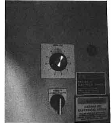
Fig. 2: An SCR type of Variable Voltage Control
